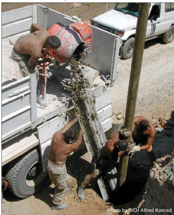
Concreting and setting snow posts, 4 soldiers of 1 st Coy
