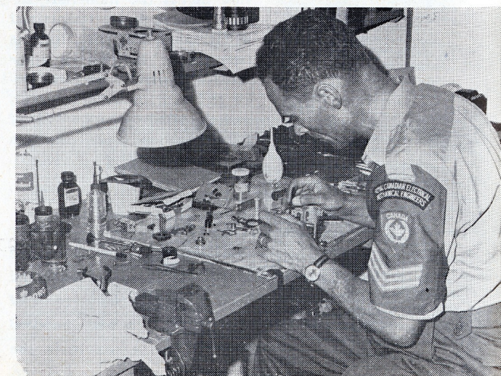
● Sergeant Stratton MacDonald, of the Telecommunications Section, at work repairing the gear box of a movie projector.
