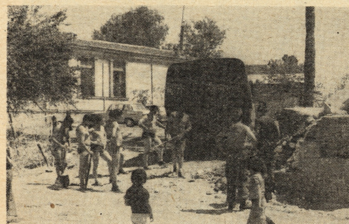
Members of 2 troop at work on project "back gate". They rebuilt the crumbled wall and constructed a new, more useful, rear gate to the Beaver Lodge compound.
