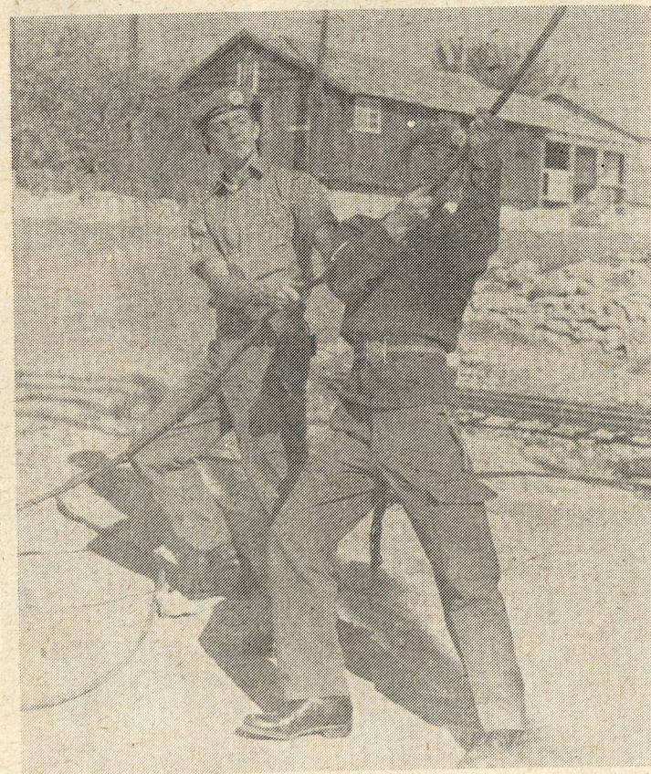
● Polemidhia Telephone Exchange operators Corporal Ricky Hassett and Lance Corporal Tony Finn haul up a new telephone cable.
