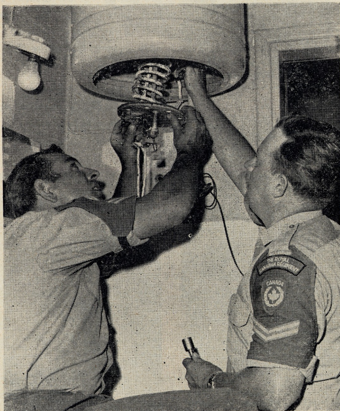
● Plumbers, Corporals "Doc" Heffernan (left) and Raymond "Magoo" McEachern replace a heating element in a hot water tank at Maple Leaf Manor.
