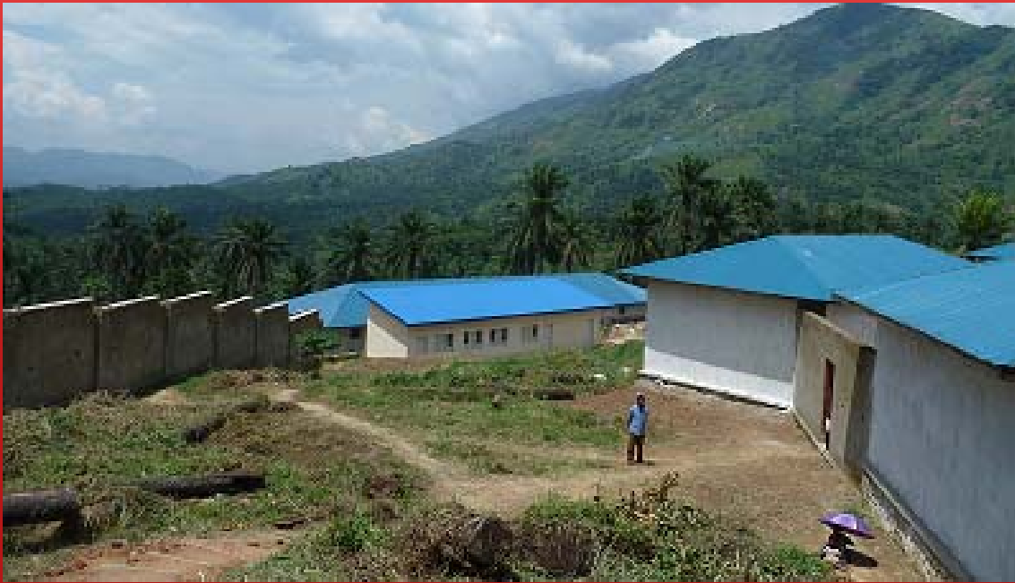
Top to bottom: Prison completed in Bunyakiri by UNOPS;
