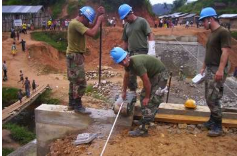
Uruguyan Engineering Company at work preparing the launching of the bridge
